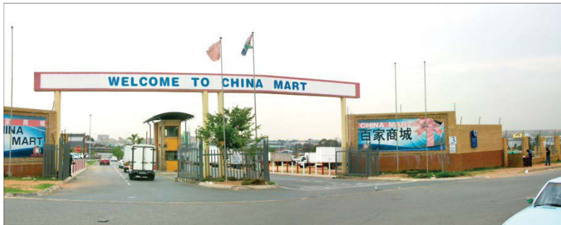
Figure 1: Entrance Gate of China Mart
